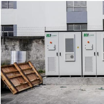
battery cabinets that may be installed adjacent to the UPS or in a separate location, are wired with external customer-supplied conduit and wiring, ...
